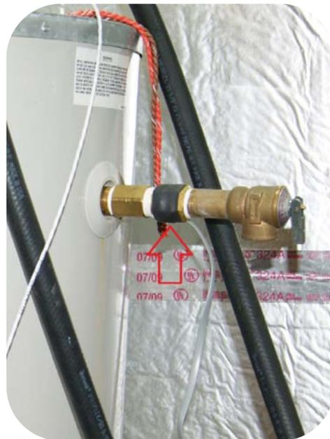
**Figure 3-2** Photo of Sunnovations, Inc. Ohm sensor
