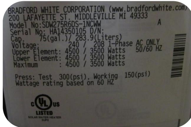
Figure 3-3 Tank label plate for **Bradford White** SDW275R6DS-1NCWW
